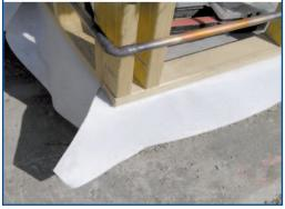
**HomeGuard DPC** (Damp Proof Course) is a tough 500 micron UV stabilised polymer sheeting containing Biflex Termiticide that offers both perimeter subterranean termite protection and damp proofing through the one installation.
