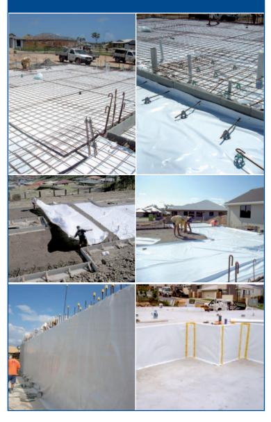
**HomeGuard TMB** (Termite & Moisture Barrier) as the name implies offers the builder both a moisture barrier and a subterranean termite barrier in the one installation. TMB is available in a  $4m \times 50m$  sheet.
